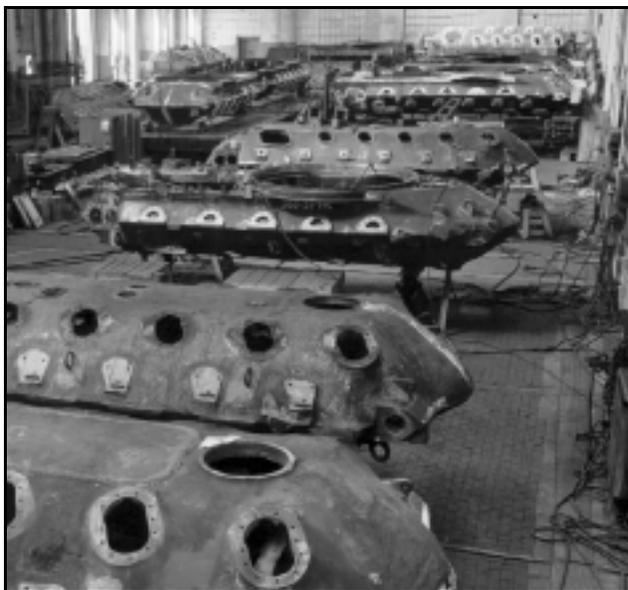
ABOVE RIGHT: In a 1952 view, bare cast hulls await installation of suspension components. Today's tank hulls are not castings, but are made up from plates of steel armor.
